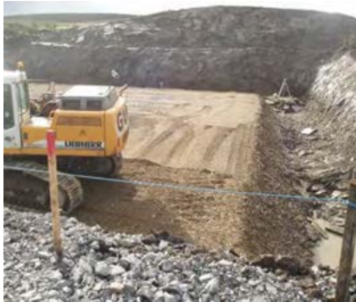
Photo 6: Excavated material stockpiled around the perimeter of the foundation excavation
