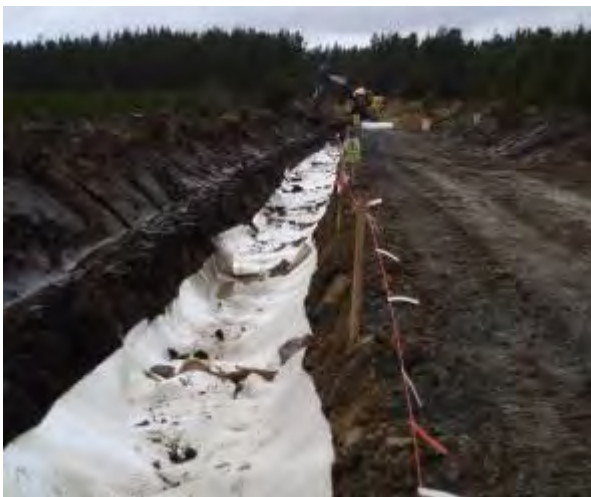
Photo 1a: Track verge reinstatement works
