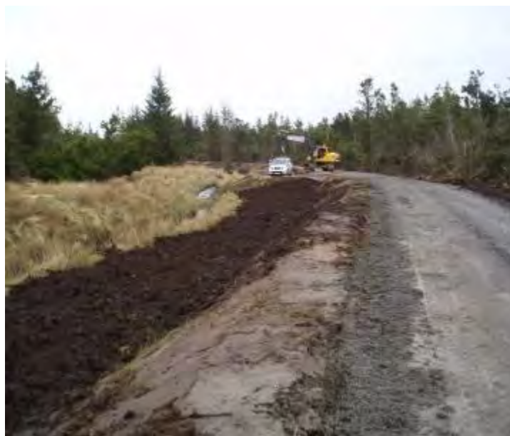
Photo 4: Example of excavate and replacement access track verge reinstatement with peat turves
