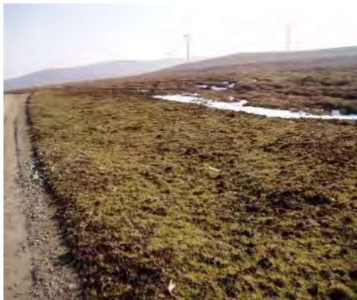
Photo 4: Example of re-seeded track verge following construction
