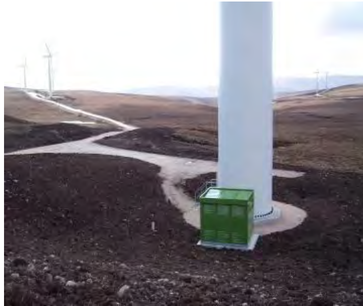
Photo 7: Reinstatement of turbine bases using excavated materials (in peat)
