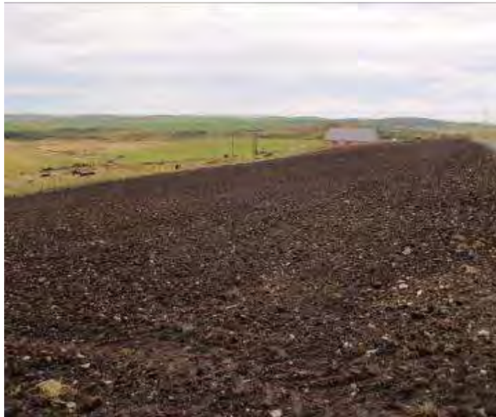
Photo 8: Example of temporary compound reinstatement
