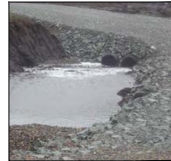
TYPICAL UNDER TRACK DRAINAGE
