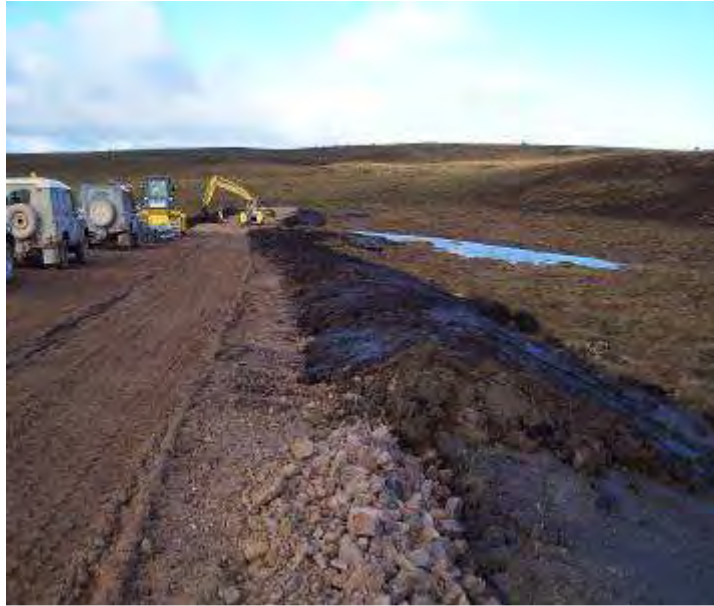
Photo 2: Example of floating track verge reinstatement whilst access track construction continues
