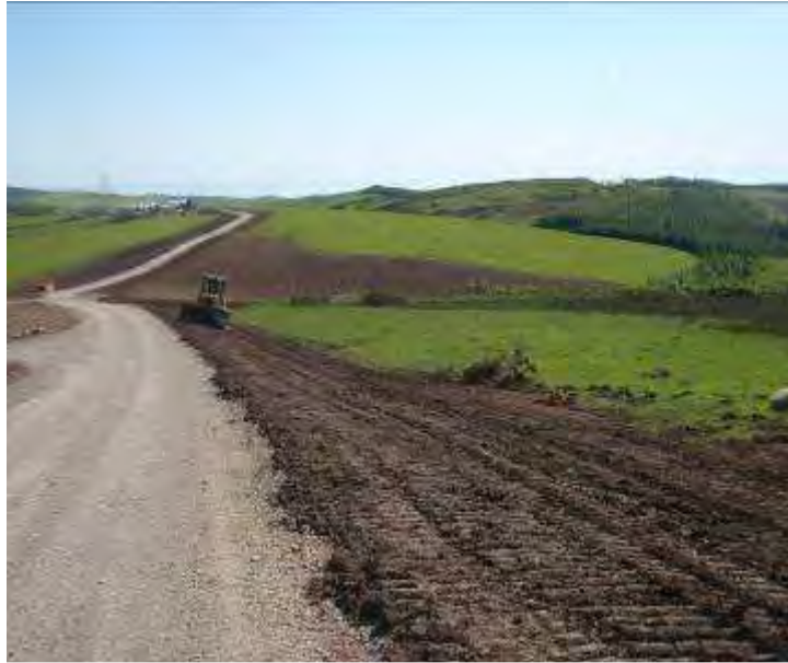
Photo 5: Reinstatement of cable trench adjacent to access track with excavated materials
