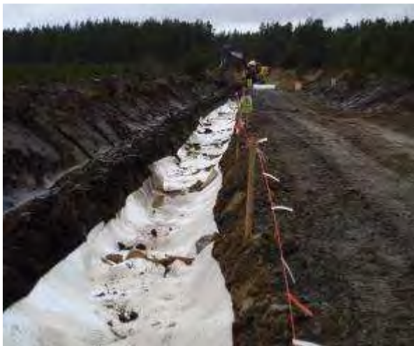
Photo 1a: Track verge reinstatement works
